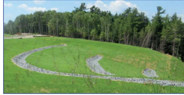
*This series of photos tells the story about the final restoration of the Landfill Ridge Area. After completing the excavation of contaminated soils from the area, engineers returned this past spring to install storm water management systems and regrade the newly restored slope. After seeding the new soil, watering crews spent the spring and early summer bringing vegetation back to the area to complete the restoration and recovery process.*
